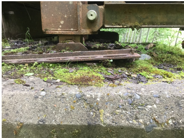
Upstream left bank bearing plate
