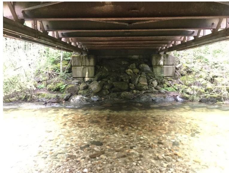
Right Bank Abutment when facing downstream
