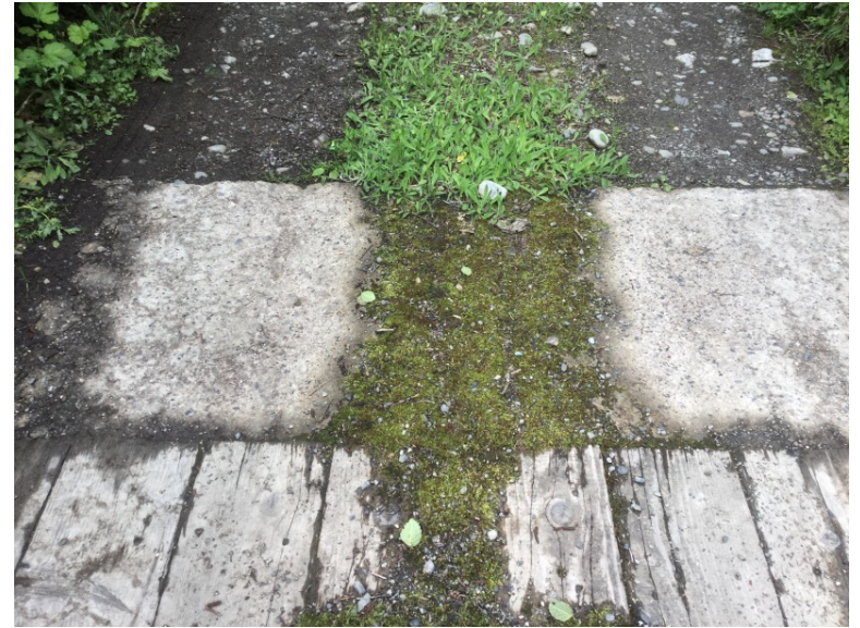
Concrete surfacing at approach
