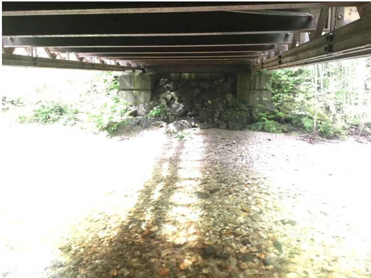
Left Bank Abutment when facing downstream
