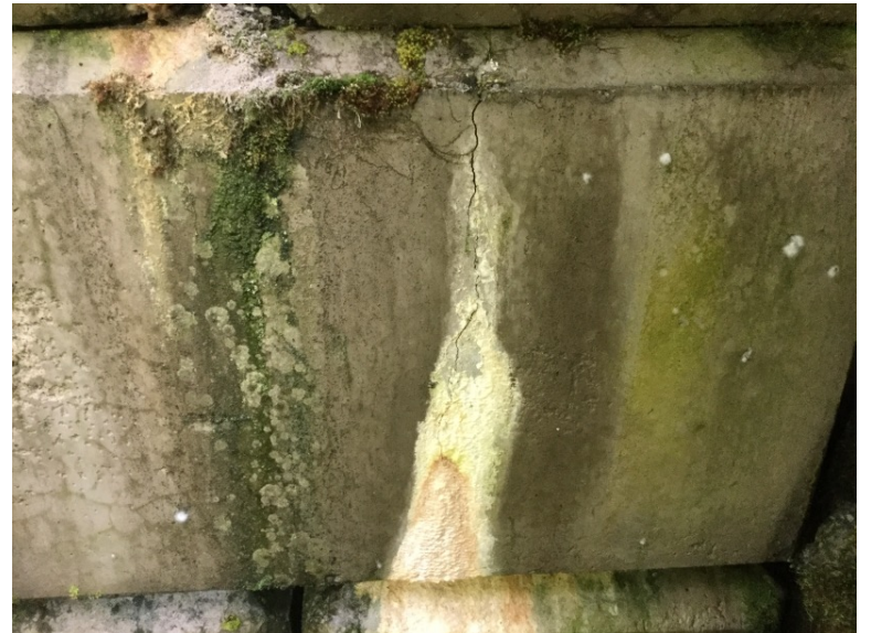
Downstream right bank lock blocks
