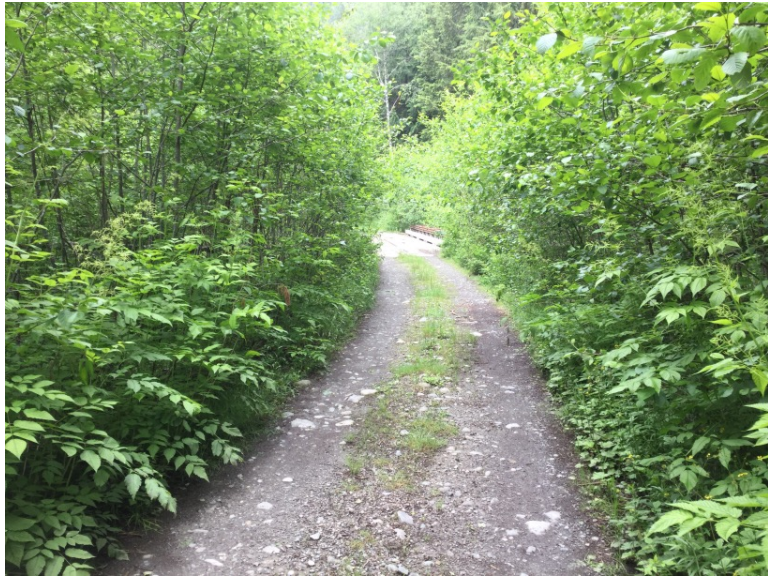
Approach from Right Bank when facing downstream
